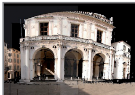
Laser Scanner FARO FOCUS 3D Rilievo Architettonico 3D
